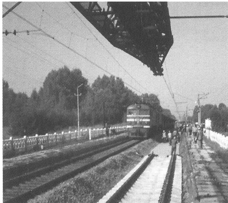
(b) Laying Track Panels with RC Sleepers
